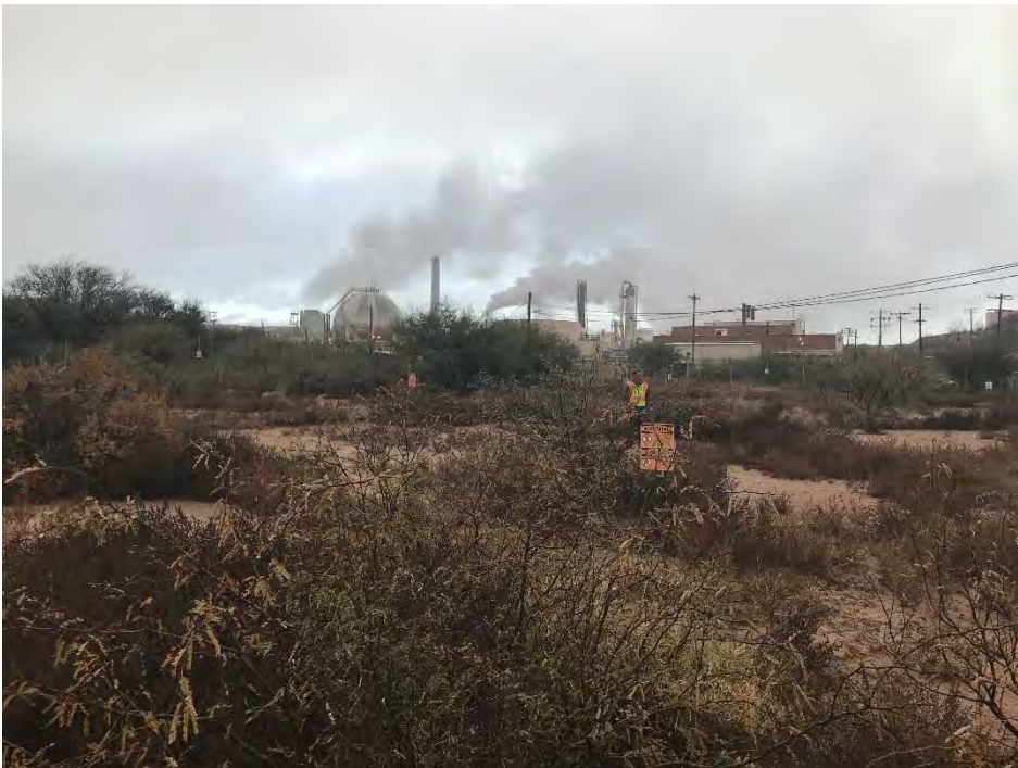
Pond 1, Looking NW 12/07/2018
